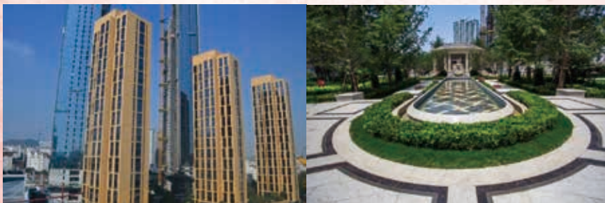
青岛悦府一期项目实景 Actual View of Qingdao City Crossing (Phase I)
