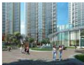
杭州悅府 Hangzhou MIXc Residence
