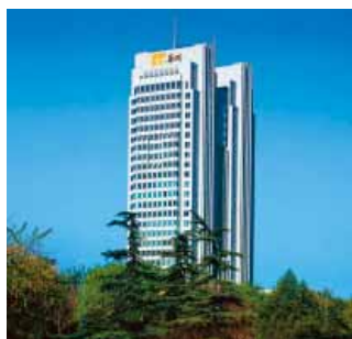
北京華潤大廈 Beijing China Resources Building
